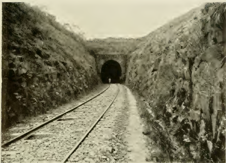
TUNNEL AT BAÑADA DE ROCHA.
